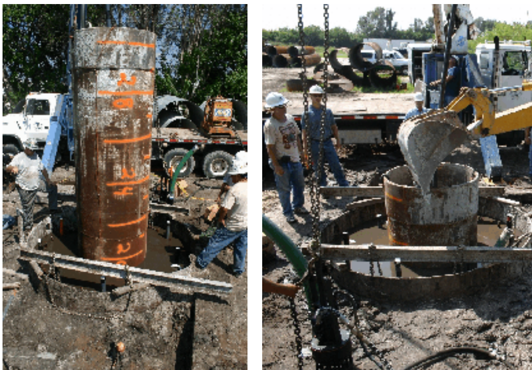
Figure 4-18. Placing and securing central casing.
