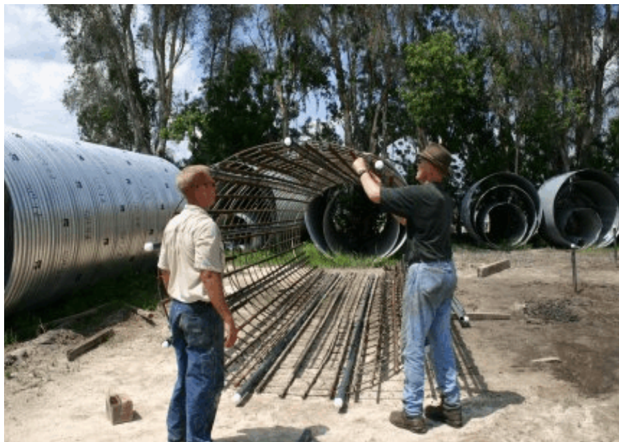
Figure 4-10. Reinforcement cage with monitoring tubes and thermocouples.
