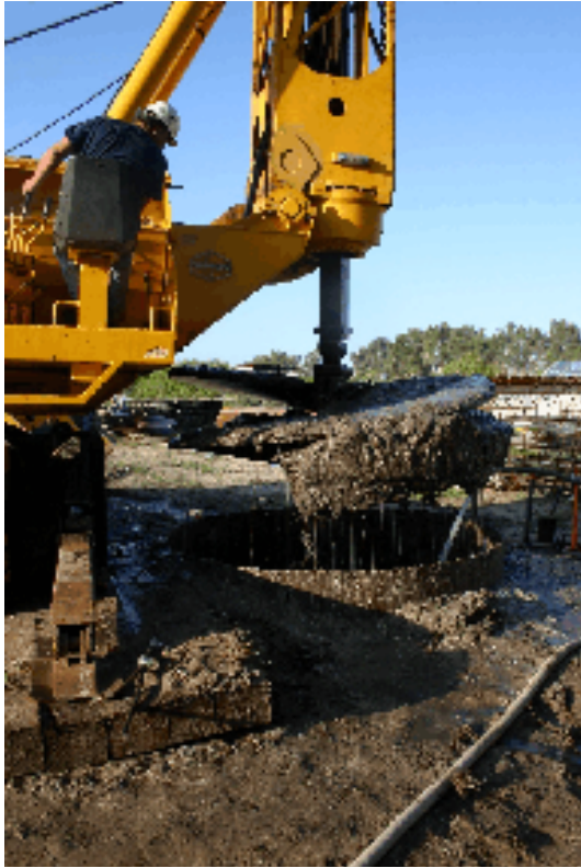
Figure 4-14. Drilling and clean-out of 9ft diameter excavation.
