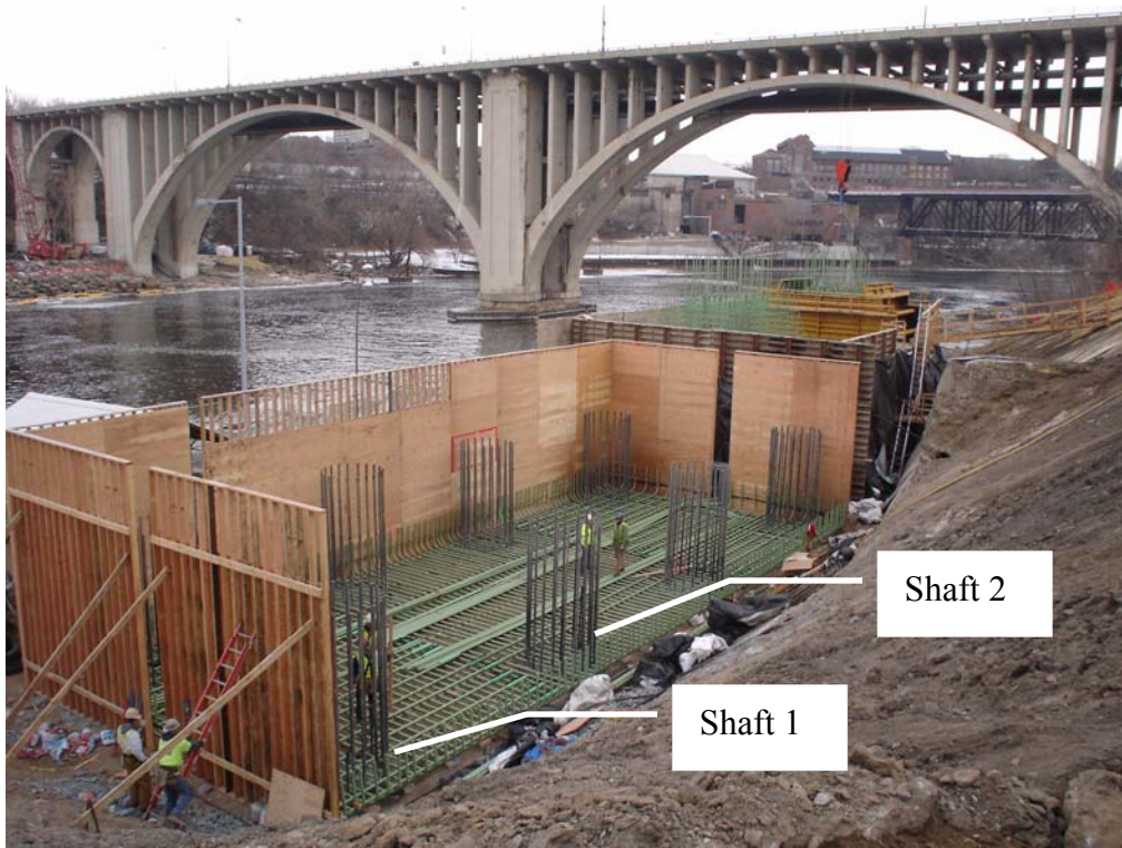
Figure 2-5. I-35W Bridge replacement southbound Pier 2 (40'x 90'x 12' \approx 1600yd 3 ).
