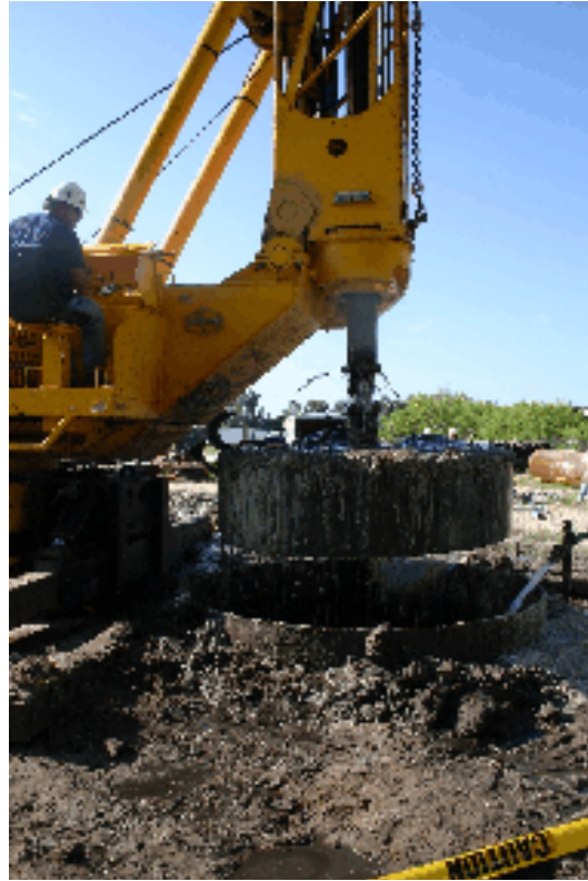
Figure 4-14. Drilling and clean-out of 9ft diameter excavation.
