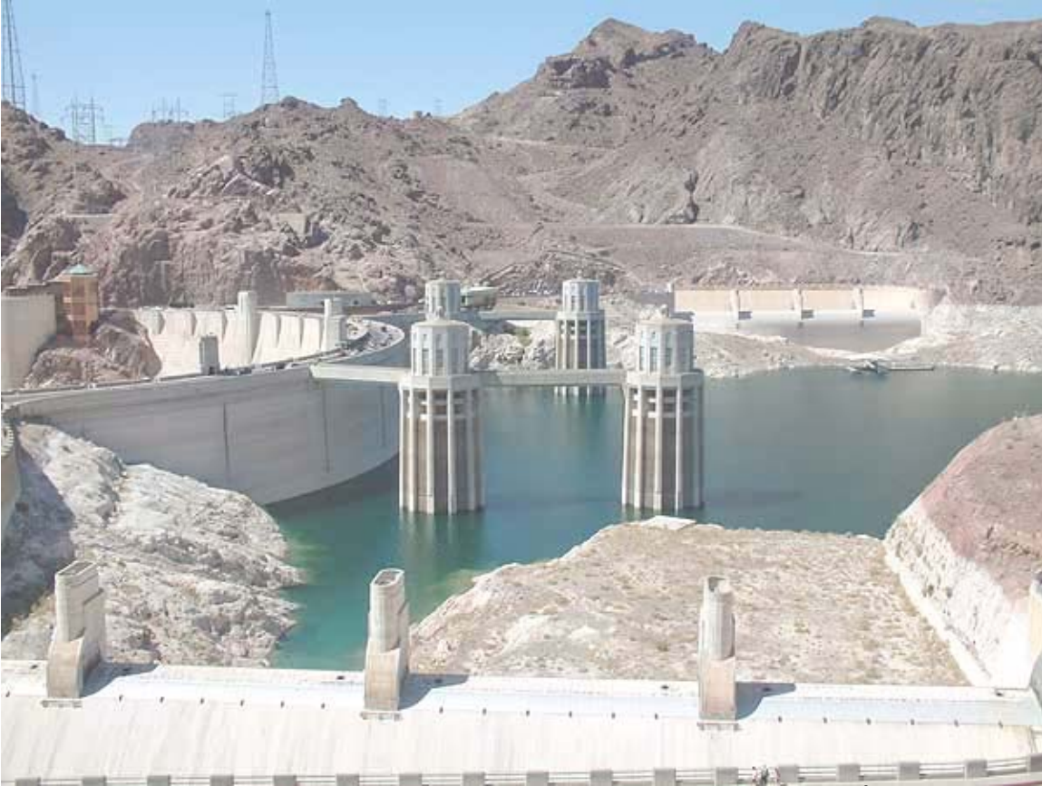
Figure 2-1. Hoover damn project (built circa 1935) used over 5 million \text{yd}^3 of concrete.
