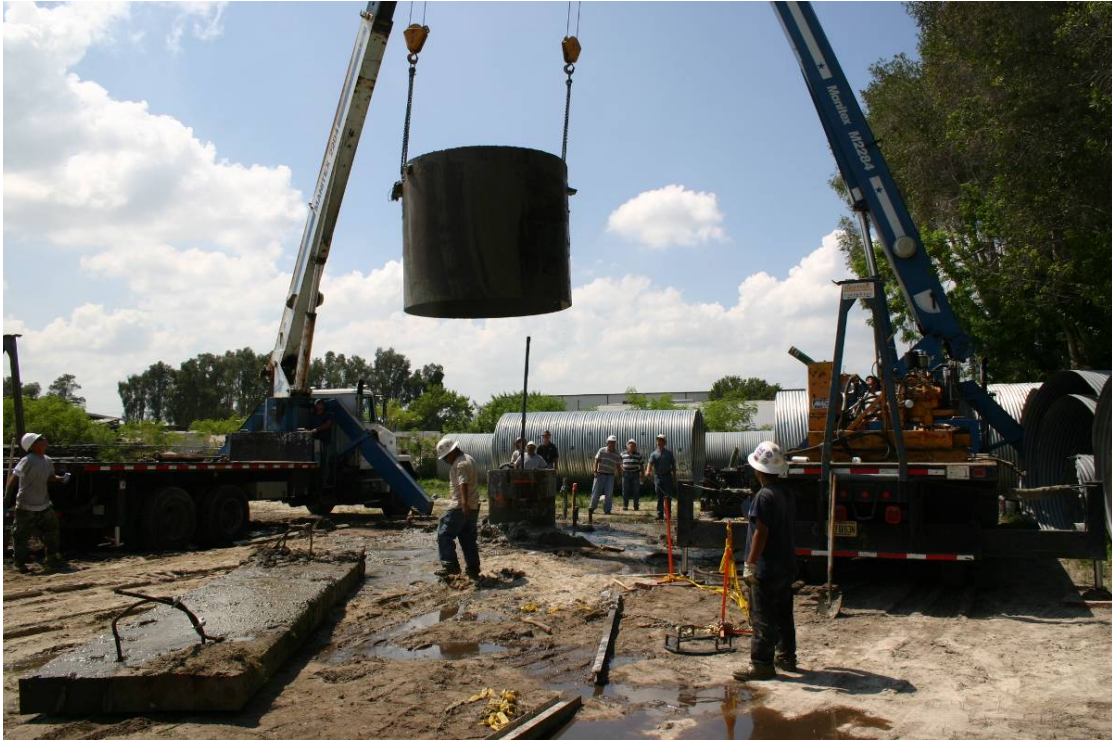
Figure 4-20. Temporary casing extraction.
